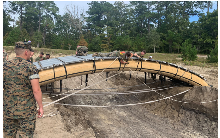
Combat Engineers deploying bridge.
