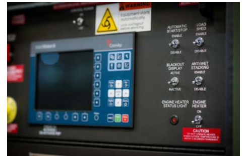
All DRASH 18 kW and 33 kW analog systems (shown above) can be converted to IPT systems, with a digital control panel (below).
