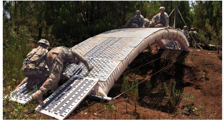
Combat Engineers deploying bridge.
