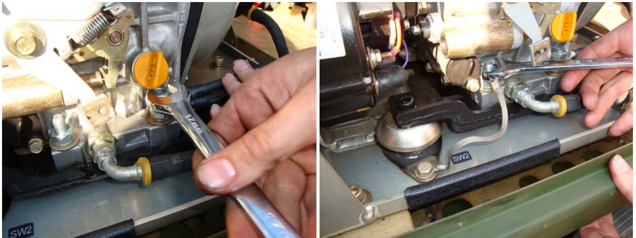
Figure 39. Install Battery Cables and Grounding Straps.
