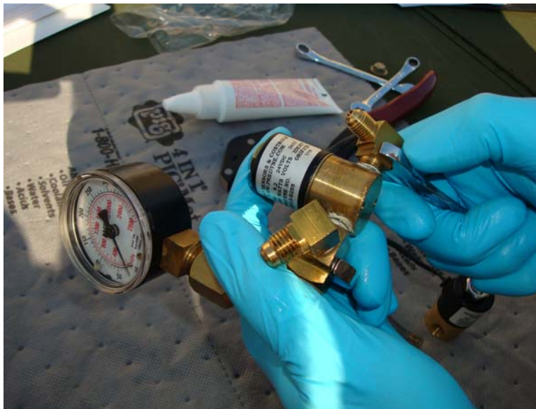
Figure 13. Remove Elbow Fitting from Side of Solenoid Valve.
