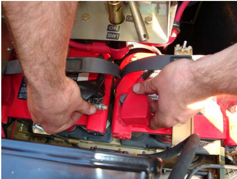
Figure 29. Install Jumper Cable Between Batteries.
