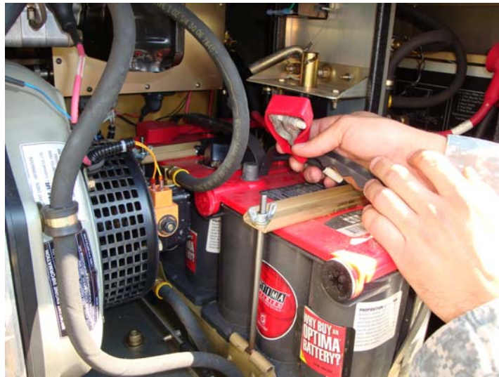
Figure 3. Remove Jumper Cable Between Batteries.
