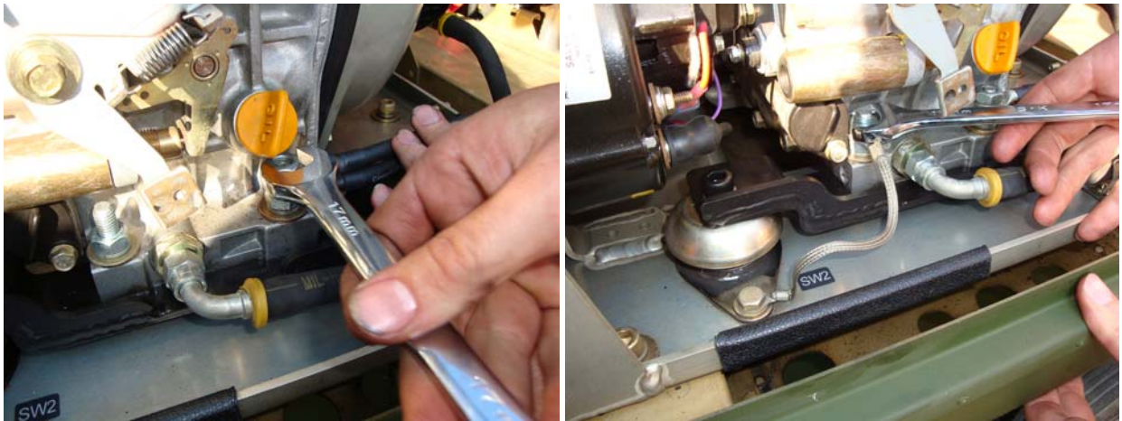
Figure 59. Install Battery Cables and Grounding Straps.
