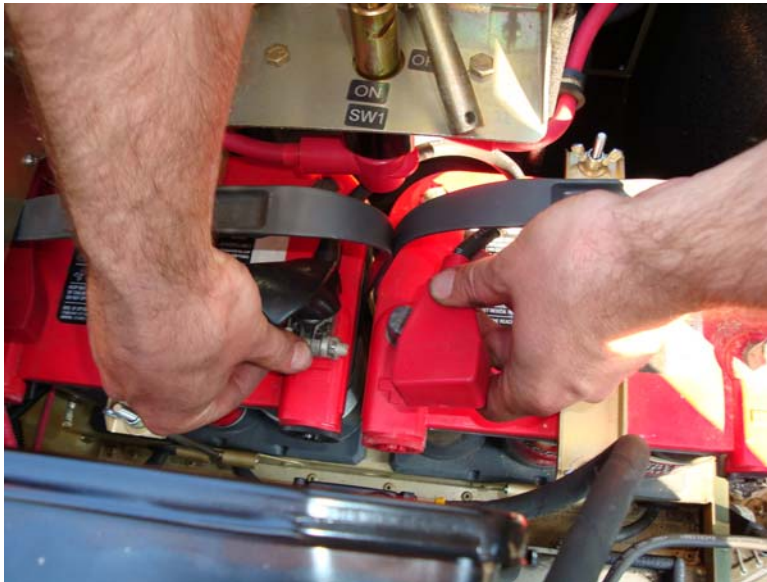
Figure 51. Install Jumper Cable Between Batteries.
