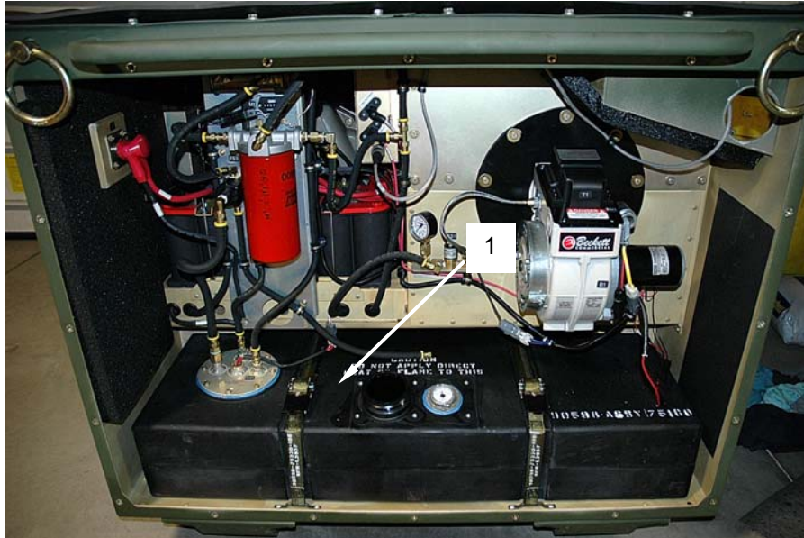
Figure 8. Repairing the Fuel Tank.
