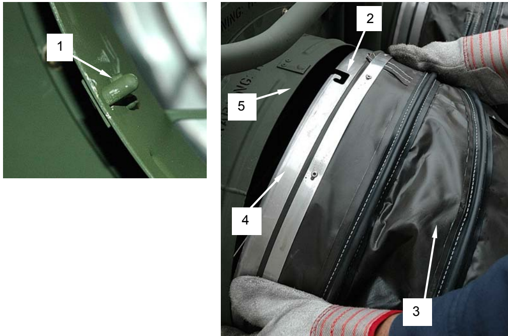
Figure 6. Install the Inlet or Outlet Duct.
