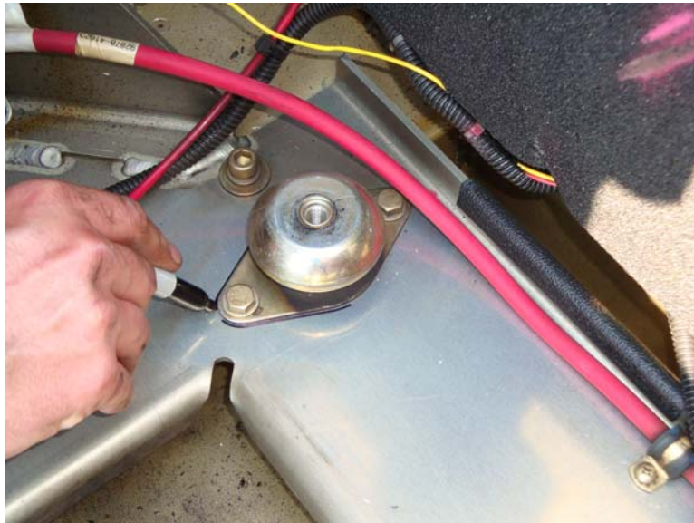
Figure 25. Marking Location of Vibration Mount.
