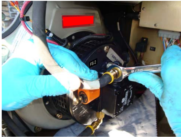
Figure 21. Reinstall Fuel Hoses onto Burner Fuel Pump Fittings.
