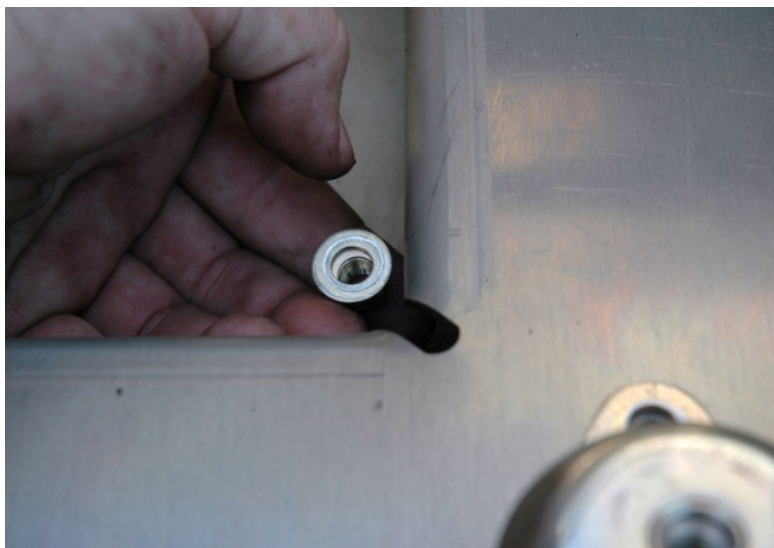
Figure 29. Installing Nut on Vibration Mount Bolt.
