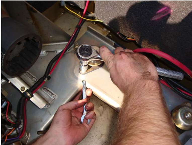
Figure 30. Installing the New Vibration Mount.
