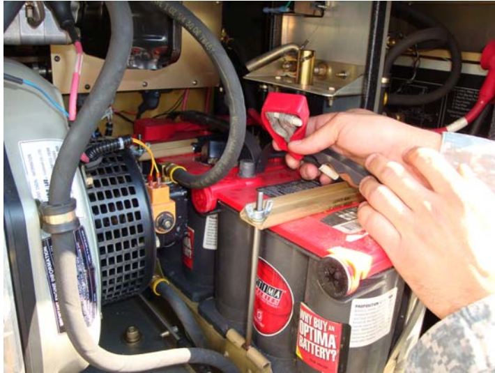
Figure 3. Remove Jumper Cable Between Batteries.
