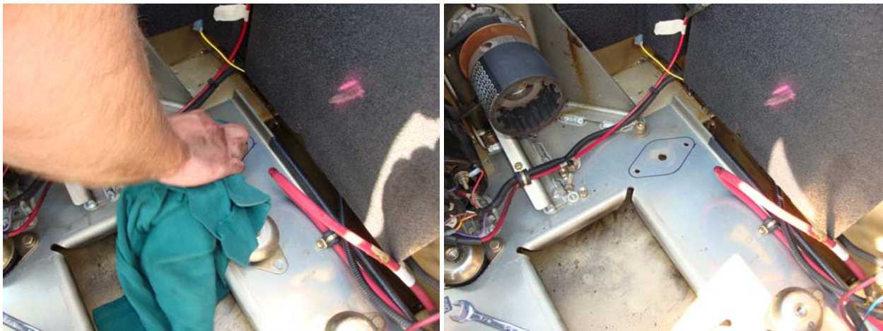
Figure 27. Cleaning the Area Below the Vibration Mount.
