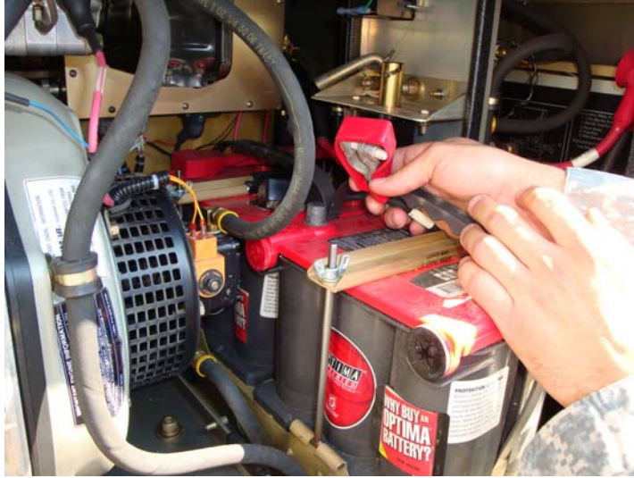
Figure 3. Remove Jumper Cable Between Batteries.
