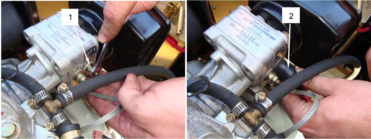
Figure 58. Install Wire to Threaded Stud Labeled GP1.
