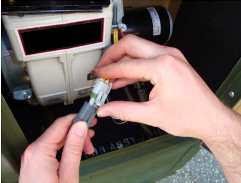
Figure 13. Disconnect Flame Sensor Connector.
