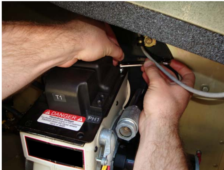
Figure 5. Position Ignition Assembly on Burner Housing and Secure with Hardware.
