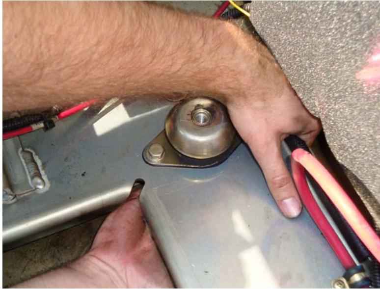
Figure 28. Place New Vibration Mount in Position and Install Bolt.
