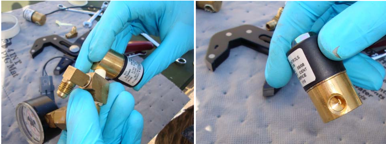
Figure 15. Apply Thread Sealant and Install Tee Fitting to New Solenoid Valve.
