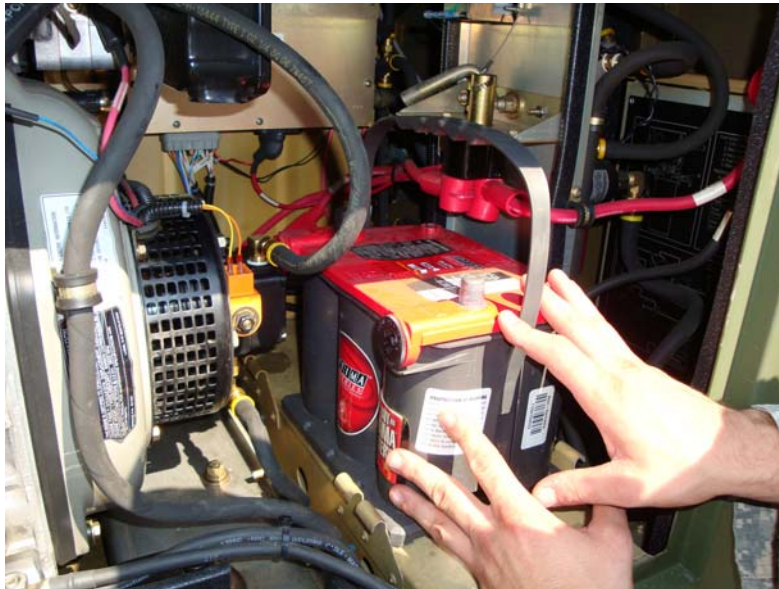
Figure 45. Install Battery Farthest from Access Door.
