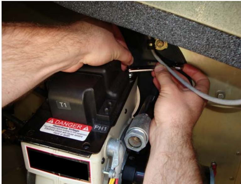
Figure 18. Position Ignition Assembly on Burner Housing and Secure with Screws.
