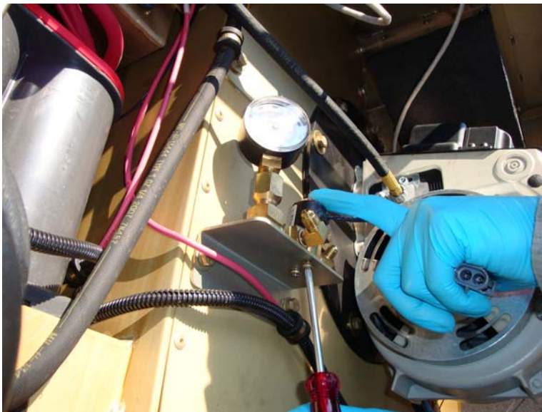
Figure 17. Install Reassembled Assembly onto Burner Valve Mounting Bracket.
