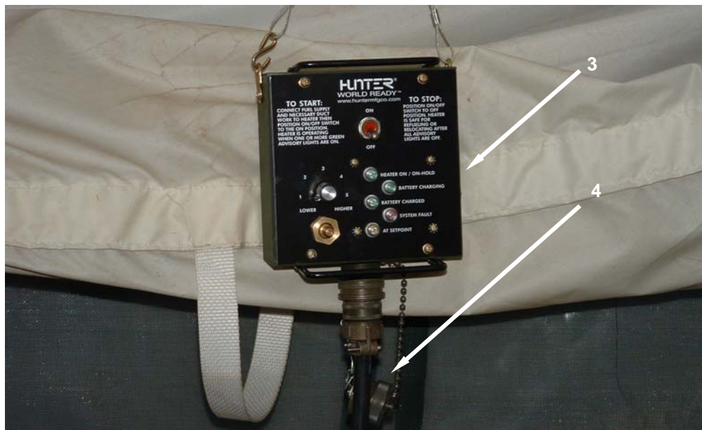
Figure 20. Prepare for Movement – Secure Duct Tunnels.
