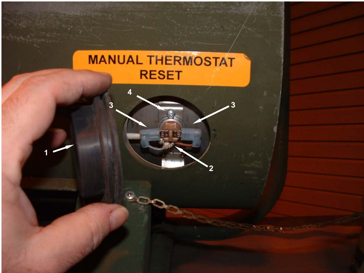
Figure 2. Replace the Manual Thermostat Reset Switch.
