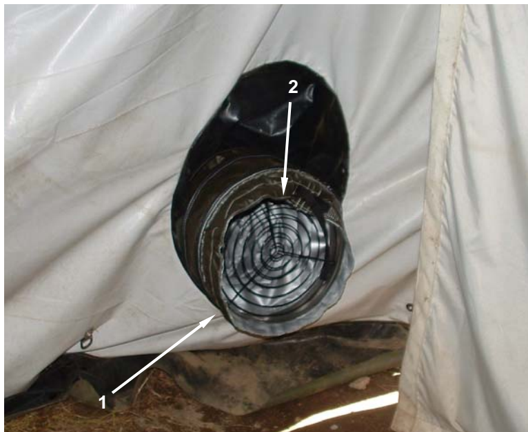
Figure 1. Return and Supply Ducts.
