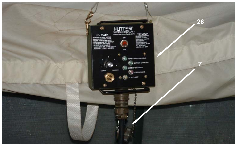
Figure 24. Prepare for Movement – Secure Duct Tunnels.
