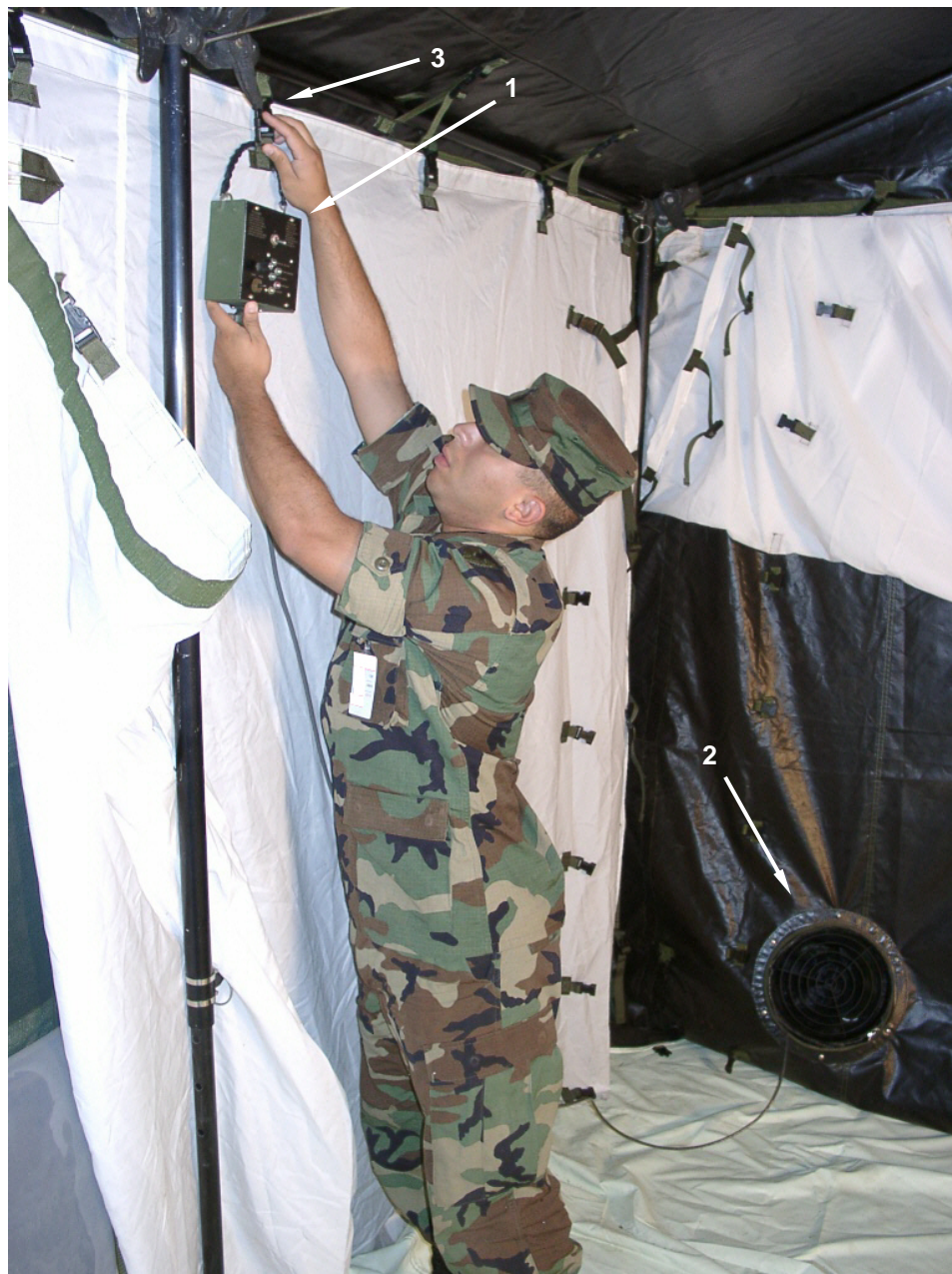
Figure 17. Positioning the In-tent Controller Inside the Tent.
