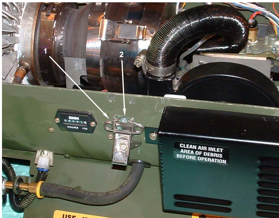
Figure 2. Repair the Lower Housing Assembly.
