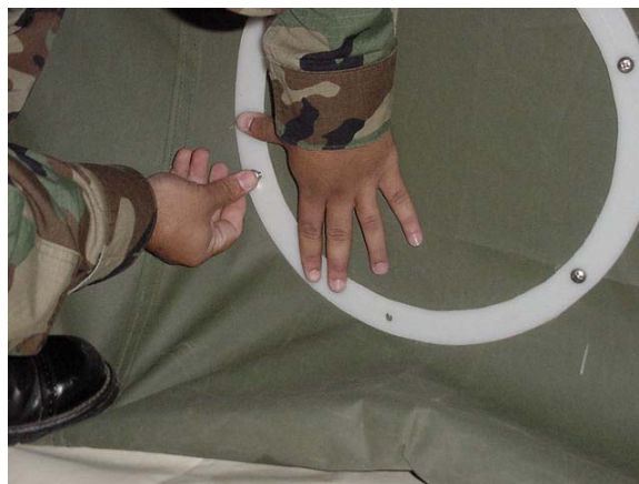
Figure 3. Locate and Begin TWMK Installation.
